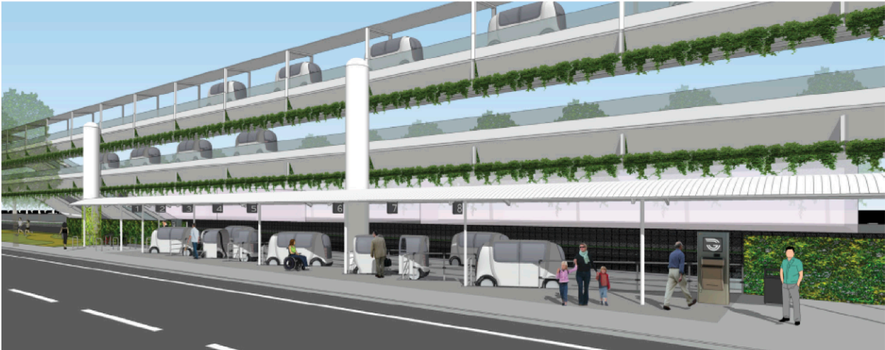
Figure C.4: Stacked Glydways guideways above a ground-level boarding station. Each guideway provides for vehicles traveling in one direction.
