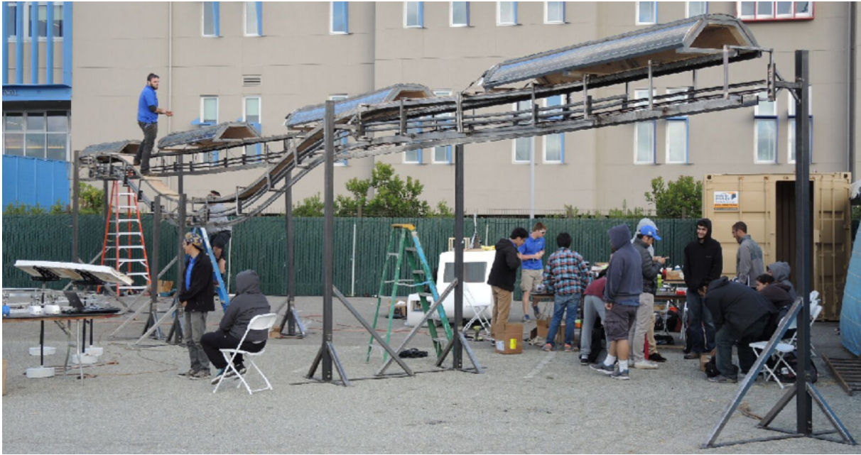
Figure 10. 2016 Half Scale Guideway. Guideway with sloped sections and solar panels at Maker Faire
