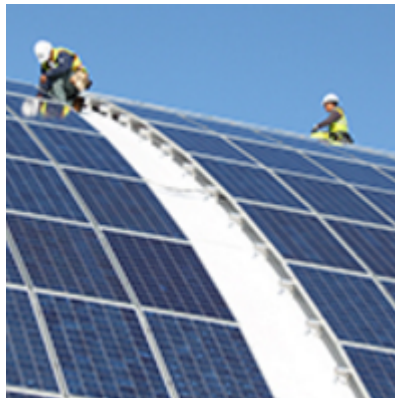
Fig 10: Standard Solar’s curved solar roof installation.
