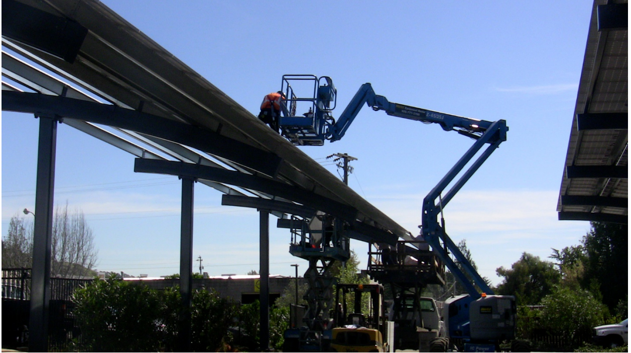
Figure 09: Module uninstalling/Installing process in the Plantronics Solar Canopy.
