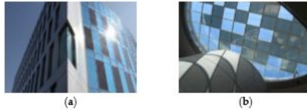
Figure 15: Example of a BIPV as solar glazing products for facades (a) and roof (b) (ASI Glass photovoltaic module, Schott Solar AG).
