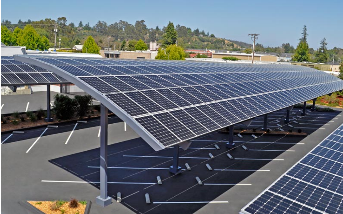
Fig 07: Solar canopy installation for the Plantronics headquarters.
