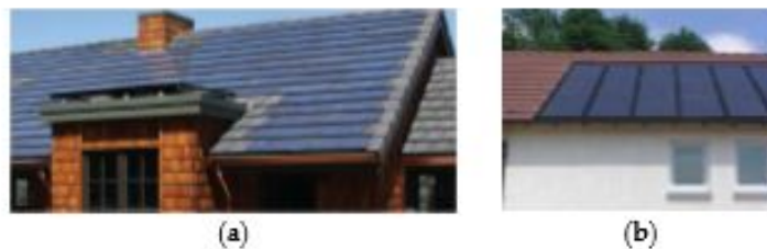
Figure 14: Examples of a BIPV tiles (a) and BIPV modules (b) (Applies Solar, DuPont)
